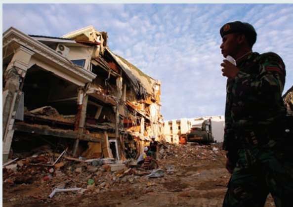
A soldier stands guard in front of the Ambacang Hotel, which collapsed during the earthquake in Padang, West Sumatra province, Indonesia, on 7 October 2009 REUTERS/Nicky Loh
